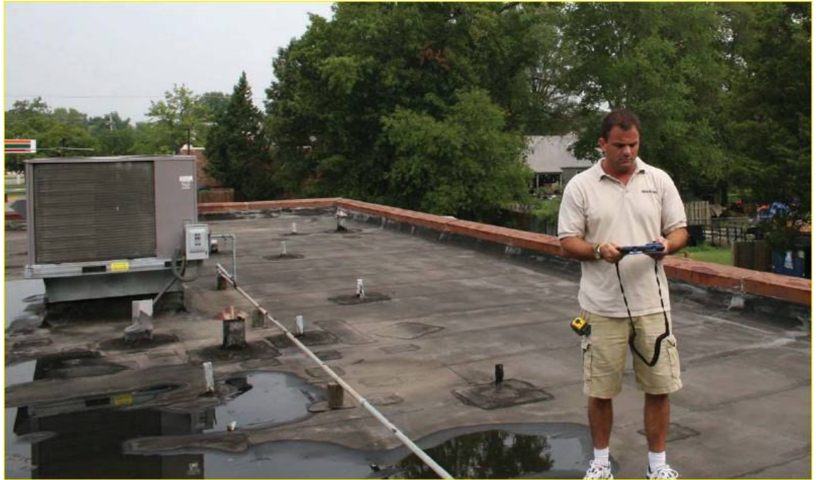
Bernie Stanley does a rooftop estimate for a client. (Contributed photos)
